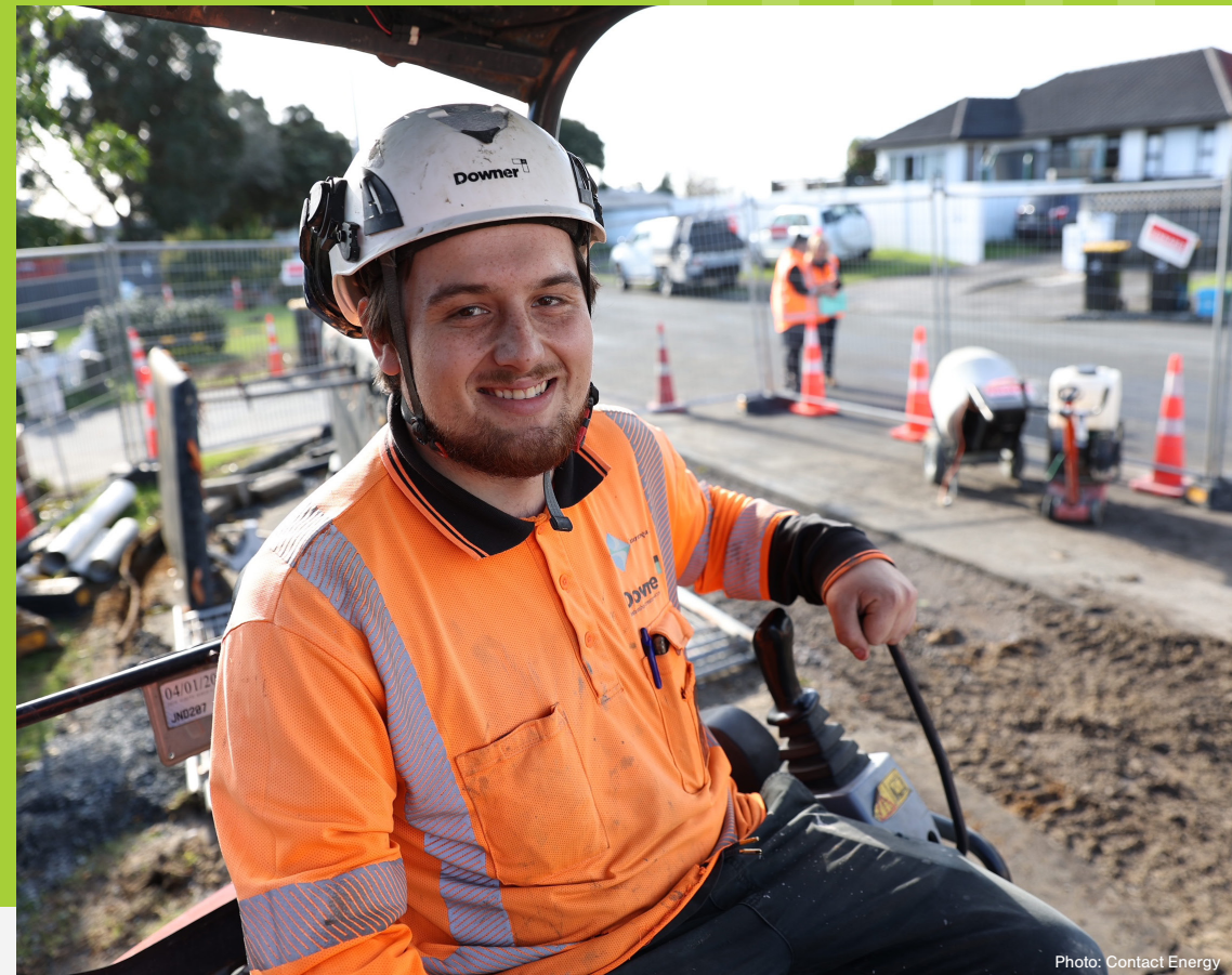
Photo: Contact Energy
