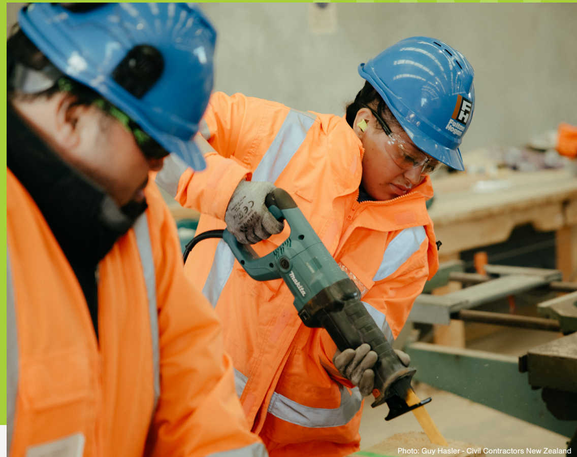
Photo: Guy Hasler - Civil Contractors New Zealand
